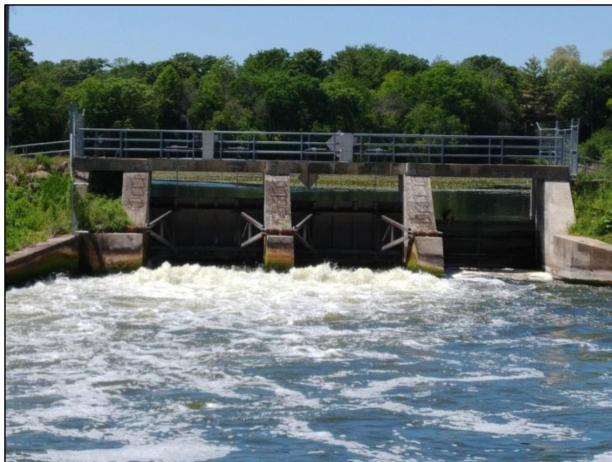
The Stoughton Dam from the 4 th Street Bridge in Stoughton, WI
