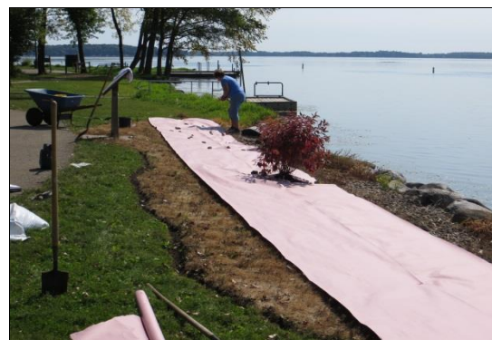
Site Preparation: Marking the site, Killing grass, Digging perimeter trench, Laying down heavy paper
