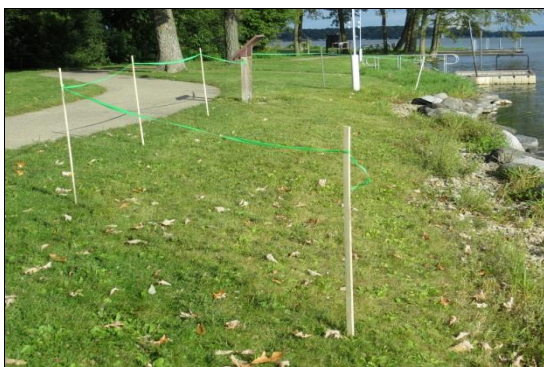
Site Preparation: Marking the site, Killing grass, Digging perimeter trench, Laying down heavy paper
